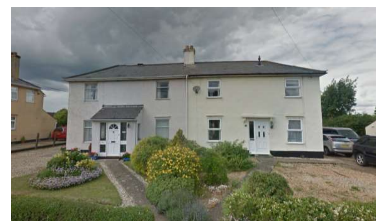
Existing dwellings on Sherman's Road
